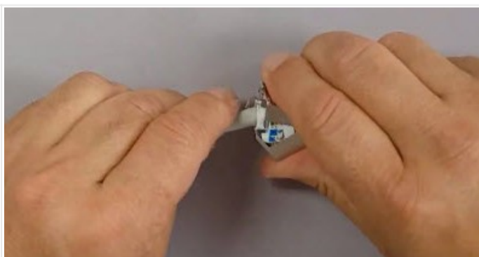
Roll back the braid or drain wire so it will fit under the jack body. Close the rear covers, pressing firmly until the jaws close and click into place
