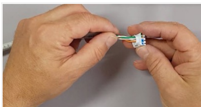
Insert the wires through the back of the wire forming cap
